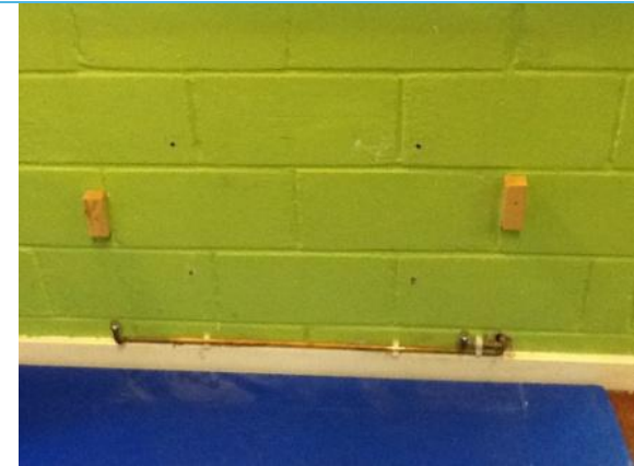
Img021: Removed Radiator
