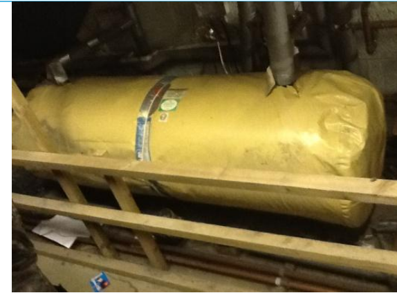
Img003: Calorifier
